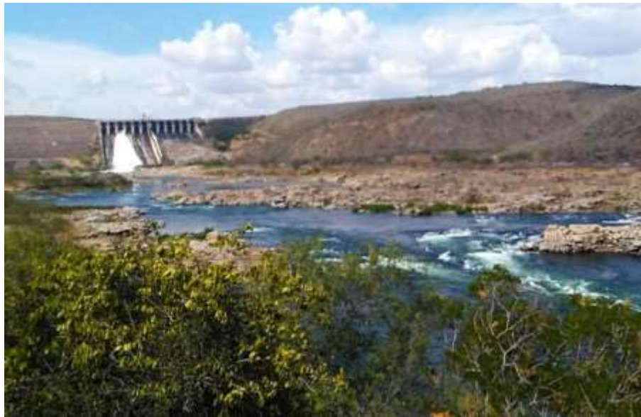
Figure 5: Xingó Hydroelectric Plant, semi-arid region between Alagoas and Sergipe States Source: Collection of the Authors, 2018.
