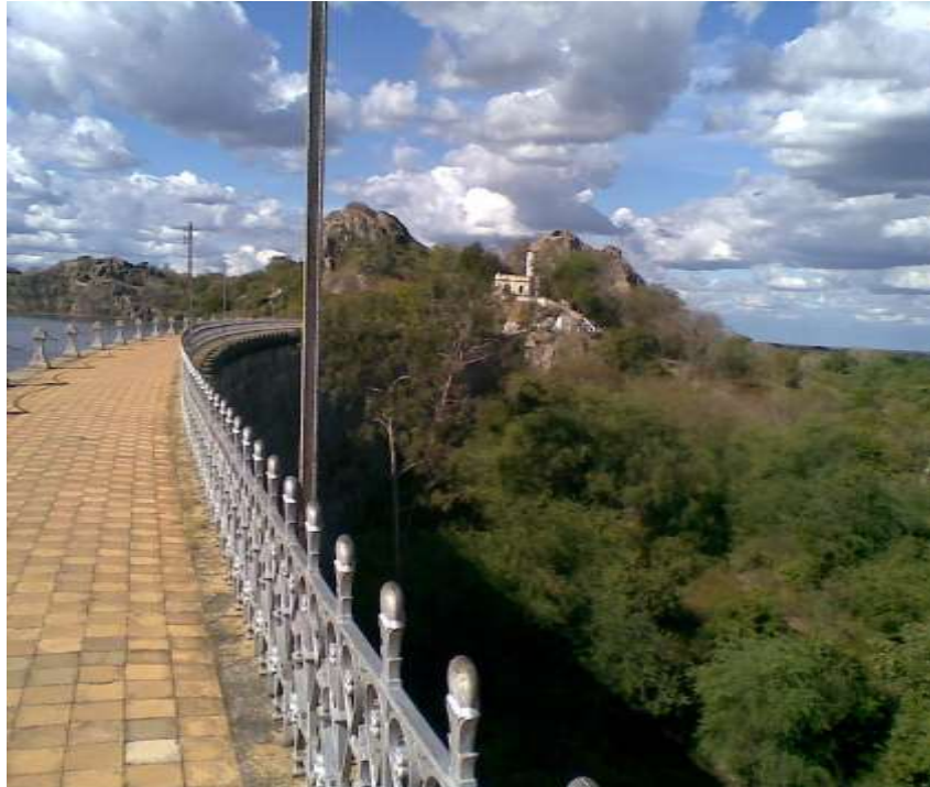
Figure 4 – The ceramic floor of the dam crest.
