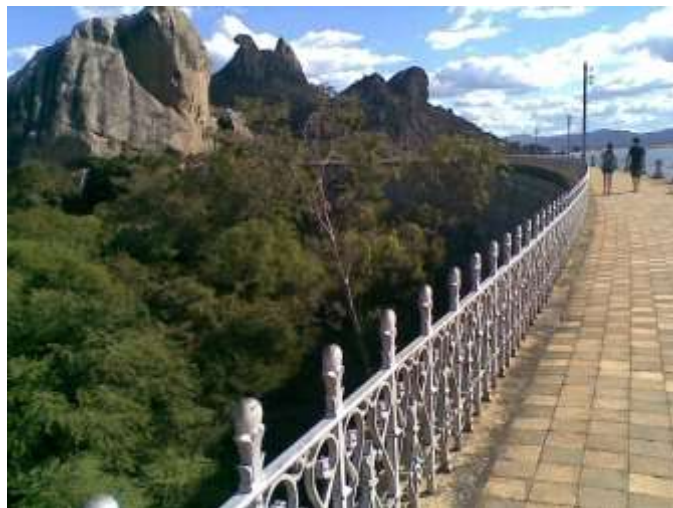
Figure 3 – End of the right shoulder where the monoliths are. The main dam is next to the monoliths.
