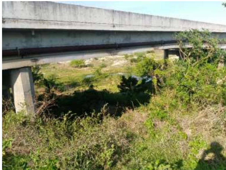
Figure 4 - Reinforced concrete bridge on the highway over the Curu River.
