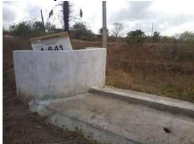
The Biodigesters generate the biogas that ensures food is cooked in the homes of many low-income families in the semi-arid region. The gas is produced from the fermentation of organic matter from animal husbandry waste. In addition to being cheap, the technique is sustainable and reduces the removal of firewood from native vegetation areas.
