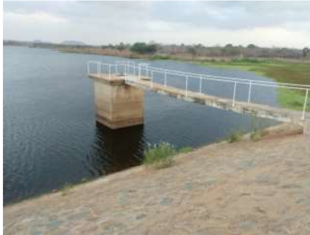
Figure 8 – Stone-lined earth dam and reinforced concrete water intake.
