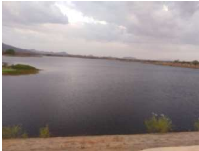
Figure 3 – Reservoir of the dam with a good amount of water.
