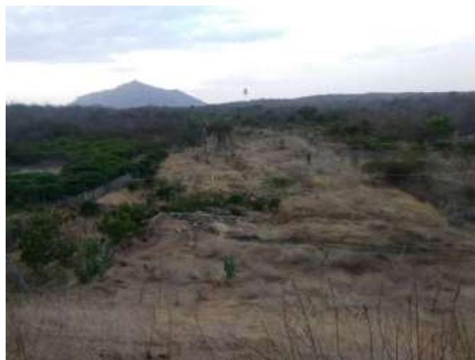
Figure 6 – Dry bed of the Aracatiaçu River downstream of the dam.
