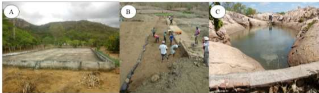
Figure 1: a) Boardwalk cistern b) Underground dam c) Stone tank
